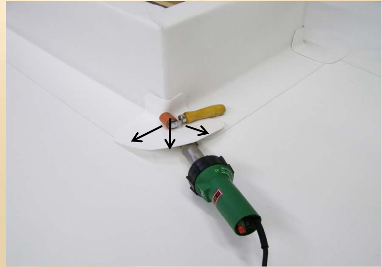
Start welding with pre-molded corner against the curb and work out onto the field sheet.
