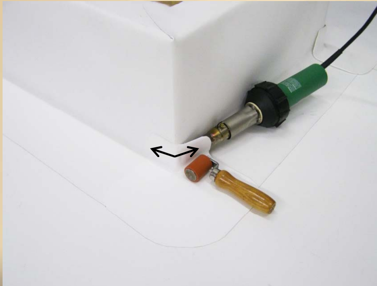
Place welder tip into vertical and work your way out.
