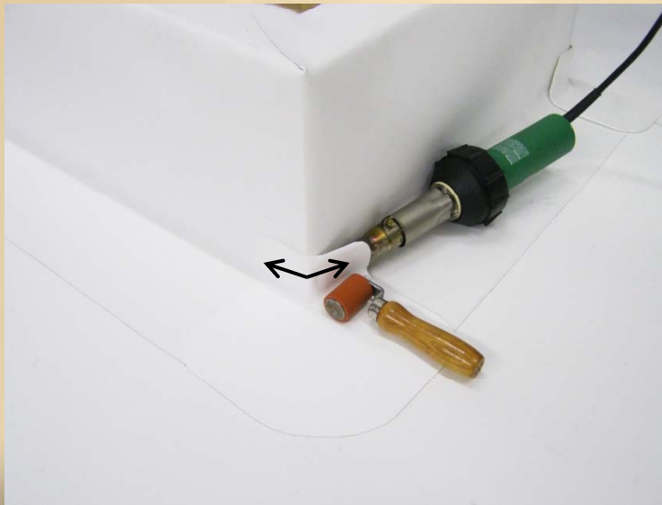
Place welder tip into vertical and work your way out. Be sure to roll the edges of the curb wrap and flashing.
