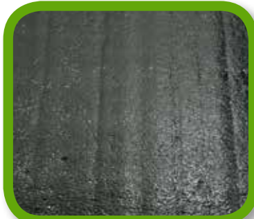
✓ Proper Coverage Uniform distribution with no light or heavy spots.
