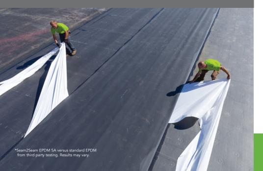
Coated from edge to edge with Secure Bond™ adhesive technology, GenFlex Seam2Seam EPDM SA eliminates the need for seam tape or spray adhesive, allowing customers to cover more roofs faster.\* Plus you can streamline inventory and optimize profitability by stocking fewer hazardous materials.
